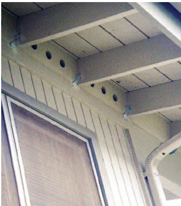
Weather-coated hurricane clips just before final finish painting.
